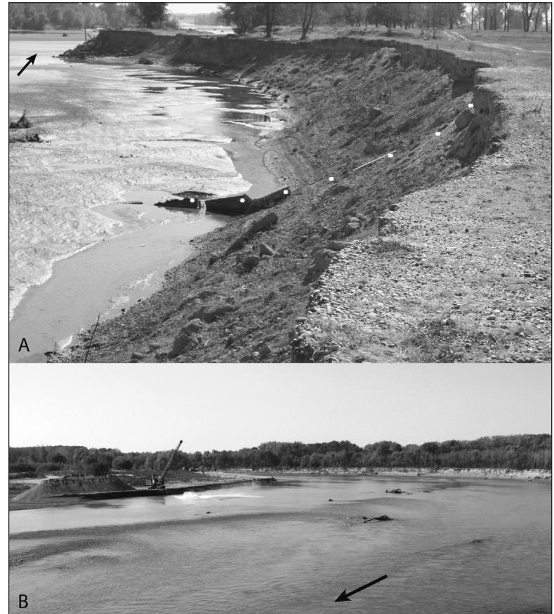
**Fig. 6 – Evaluation of the lateral erosion in the Lower River Siret by quantification of destroyed groynes.** (A) Note the seven fallen blocks (14 m) pointed by \*. (B) In-stream mining in the active channel of the Lower Siret River. Photograph: F. Salit, October 2011.
