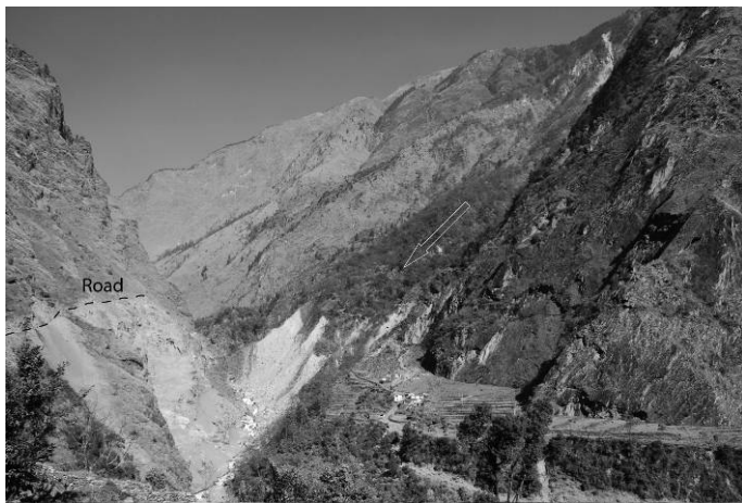
Figure 2. The Talbagar debris slide/avalanche failure, and associated sedimentary wedge downstream (right), viewed from the right bank of the Kali Gandaki river. Note the track of a new road completed in March 2008 (MF.07-02-473).
